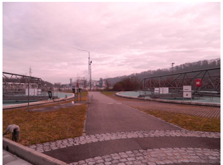
Photo 4. Main Sewage Treatment Plant of Stuttgart
